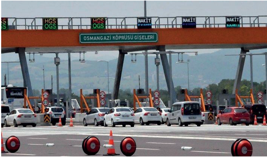
Figure 16. ETCS gate in Osmangazi Bridge
