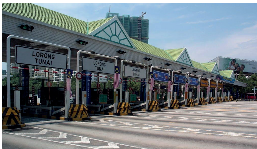
Figure 49. ETC Application in Malaysia
