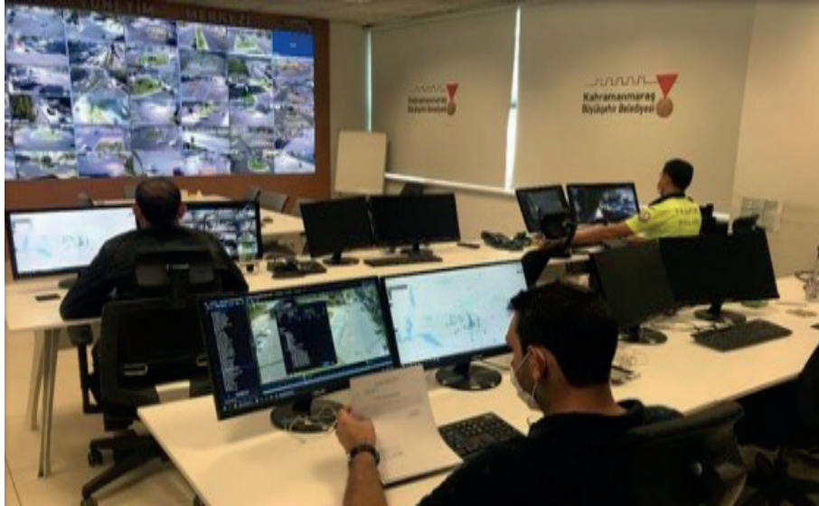
Figure 22. Kahramanmaraş Traffic Management Centre (Source: Ministry of Transportation and Infrastructure)
