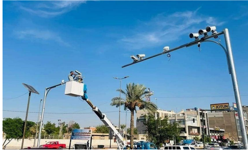
Installation of Monitoring Equipment in Baghdad (Source: Iraqi News)
