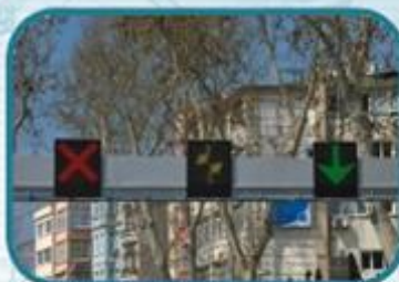
Lane Control Systems (LCS)
